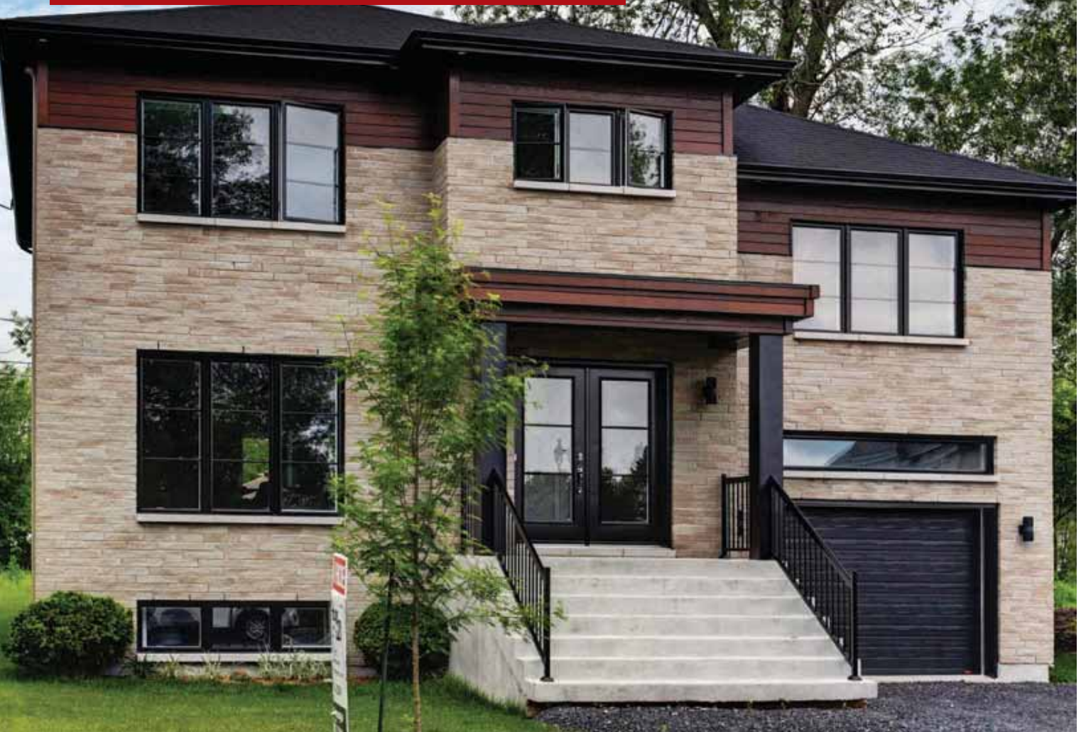
Contemporary Brick Phoenix
